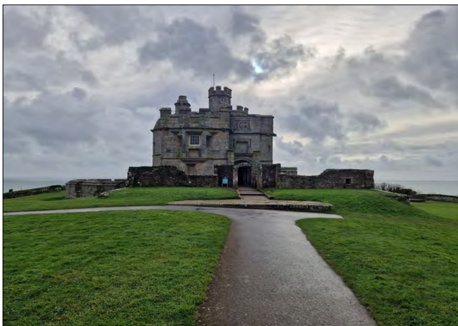
Plate 2) View of the Grade I Listed Pendennis Castle (NHLE 1270096), facing south
